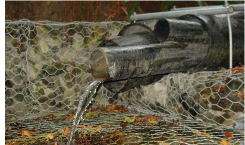
Stormwater discharging from a pipe outflow
