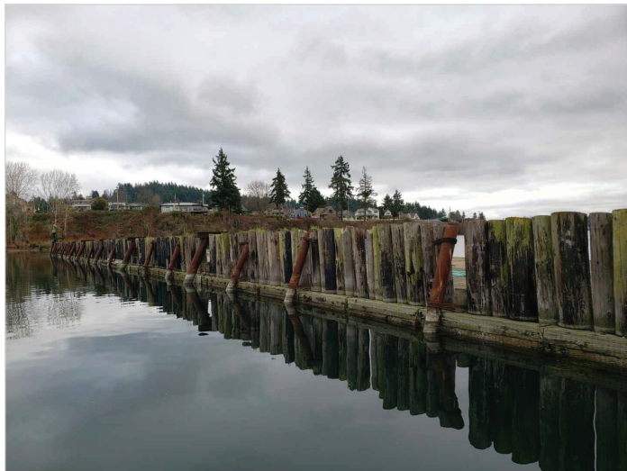
SOUTH BREAKWATER (A)
