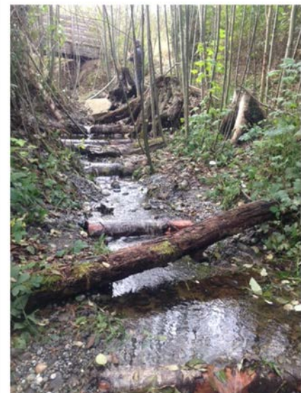
Stream restoration for SF Dogfish Creek at Poulsbo Fish Park
