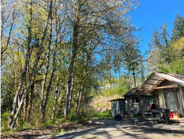
Photograph 1. Existing Residence on central parcel, view to the northwest, on April 17, 2025.
