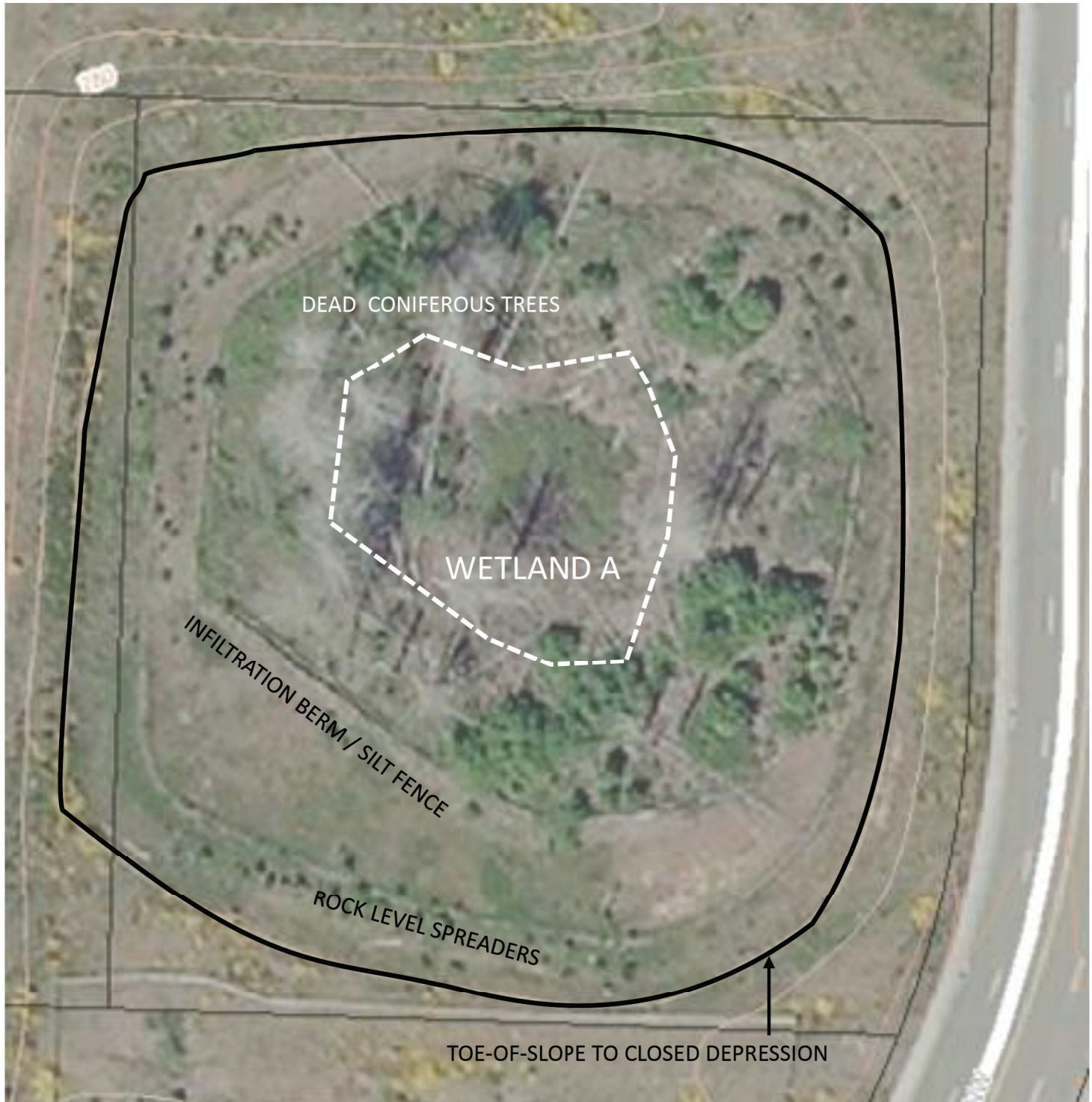
EXHIBIT C: OBSERVED CONDITIONS OF CLOSED DEPRESSION
